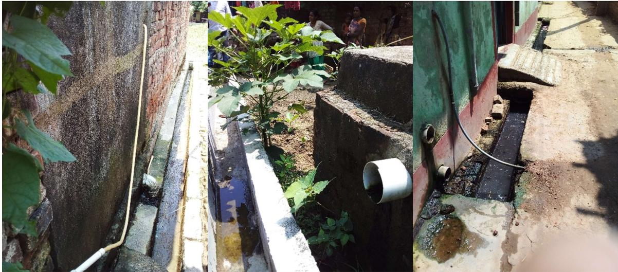
16. Village drainage system. All shorts of issues. One said that their drainage dispute with *gotia* (near relative uncle) is going on since their grandfather time. Drinking water nal-jal supply is next to open drain, hand pump is very next to open drain, septic tank effluent is discharged in open drain, solid waste accumulates in open drain, slope in wrong direction, branch drain could not be connected to main drain, drain is broken and water is leaked in near by field, keep on writing...
